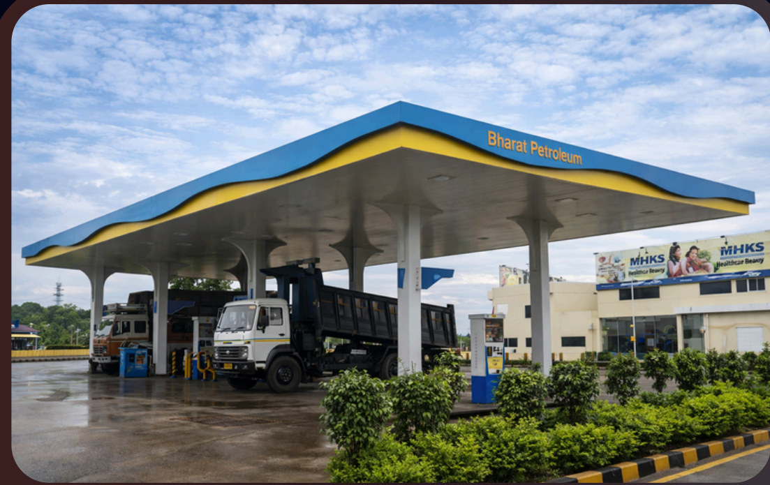
Fuel Station Canopies
